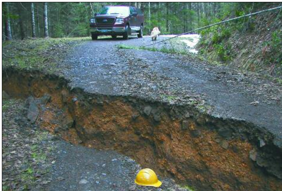
This road was built atop old logging slash and slumped during a wet winter.
